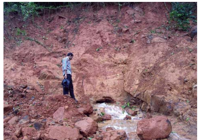
Fig. 2. Water discharge point of a subsurface tunnel at a landslide scar (Valamthode, Wayanad).
