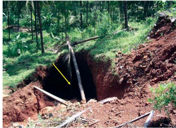
Fig. 1. Opening of the tunnel due to subsidence.
